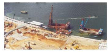
Due to the high water table, different sections of the tunnels were designed as either founding on rock via diaphragm walls or "floating" where rockhead was deep. Both "top down" and "bottom up" construction methods were employed.
