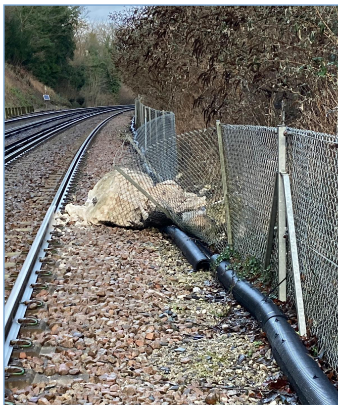
Figure 1: Fences and barriers do not always prevent falling material reaching the track
