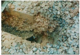
Figure 2: Severe subgrade erosion
