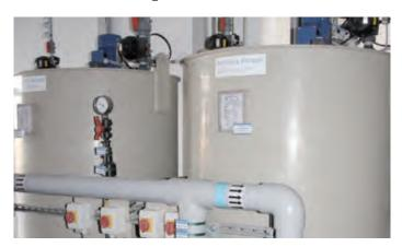
The wastewater toilet tanks of the aircraft have to be flushed with a disinfectant solution ("blue water"). The preparation of blue water is done by using a concentrate and fresh water.
