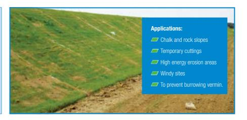
Rockmat provides a highly effective anti-vermin protection layer where rabbits and foxes, etc., are likely to create slope instability due to burrowing. Rockmat is available with coir fibre or coir/straw fibre matrix or F3. Coir fibres will last 3-5 years.
