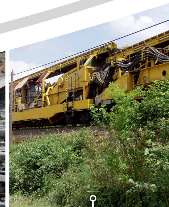
6 - Large worksite with moving track construction machinery
