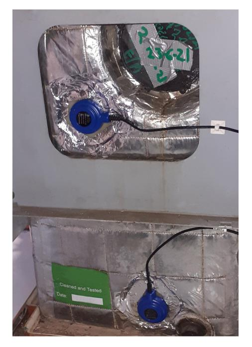
the sensor can integrate with the control systems. Most of all, Gobius technology solves the longstanding problem of overfilled waste tanks, in a smart and simple way.
