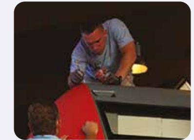
Step 9: Spot repairs of paint damage.
