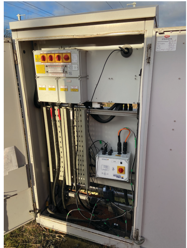
Temporary installation of roaming CableGuardian unit, which also offers the flexibility to be fitted upside down if needed. No special requirements for installation.
