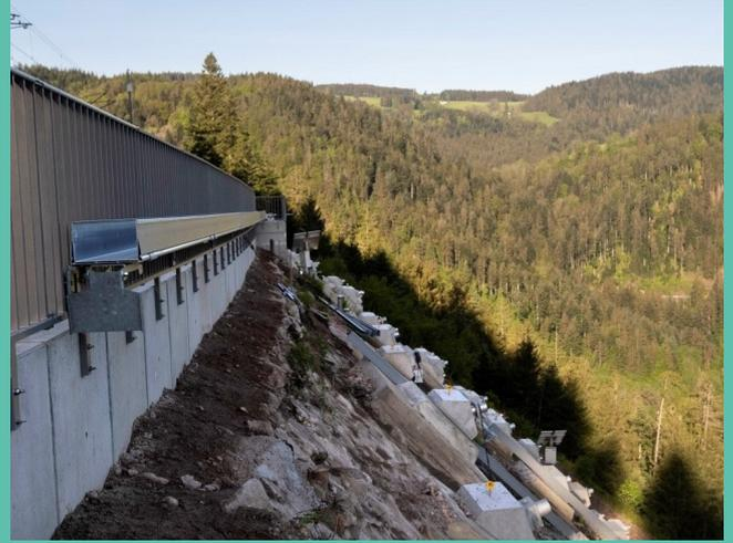
The composite troughing can be fastened to a variety of trackside structures, such as ballast boards and railings here during an installation in Germany's Black Forest
