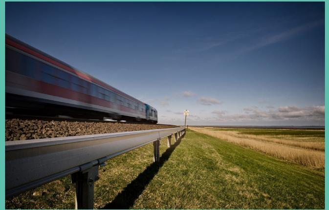
The twin-walled design of the troughing enables the system to resist lateral forces such as wind effects from high-speed trains
