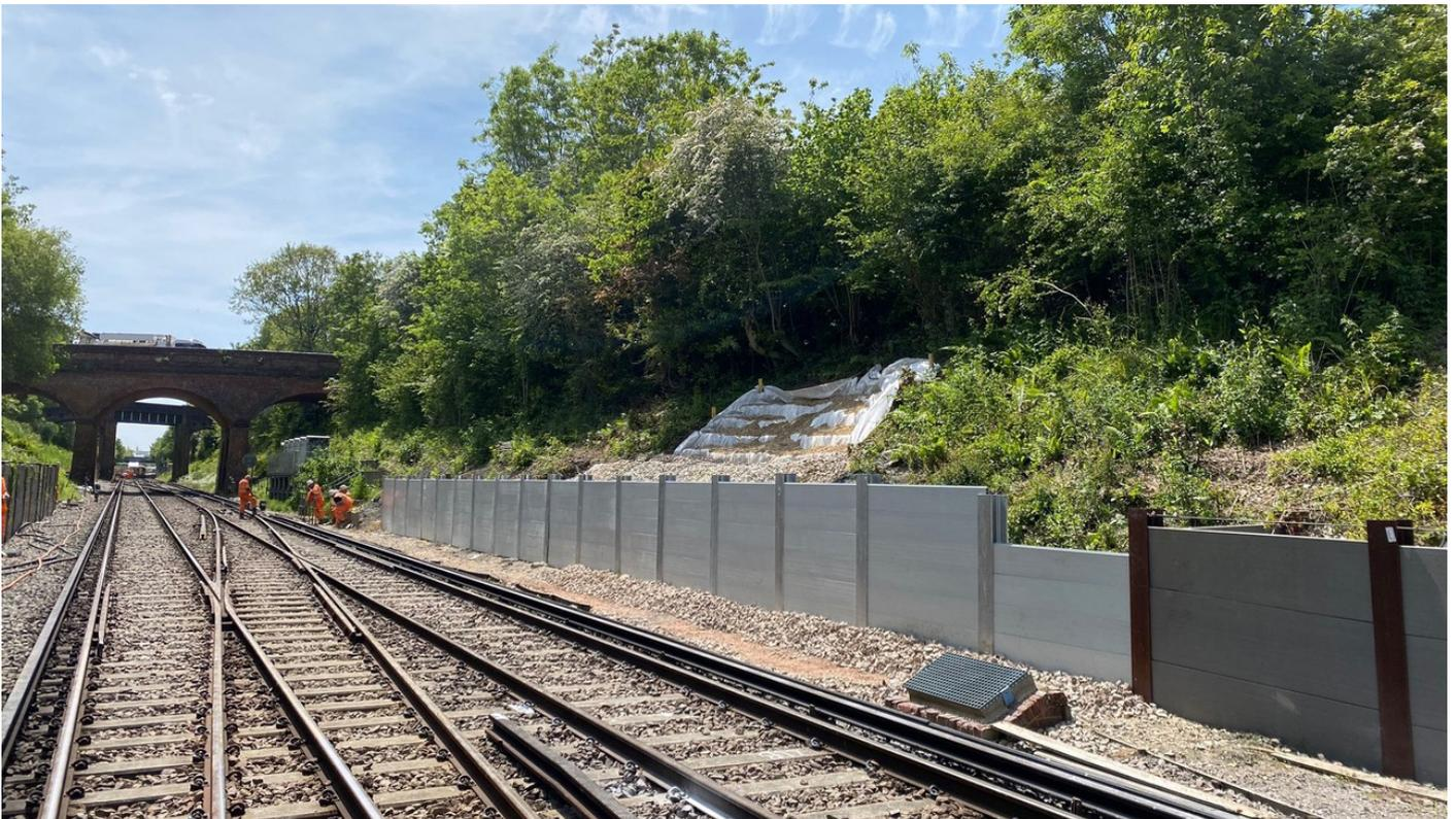
*Composite ballast boards from CCS being installed on site*
