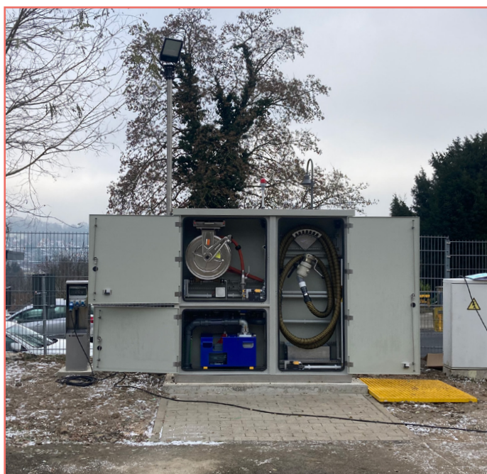
Stand-alone supply & disposal cabinet installed at Nidda Railway Station, Germany
