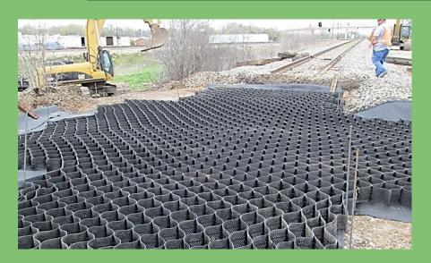
Offering the ability to repair washouts and address localised track issues quickly and economically with a single solution, the GEOWEB geocells have gained acceptance by the rail industry as
