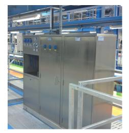
Utility Cabinet for the interior cleaning of trains, using hot & cold water and cleaning agents
