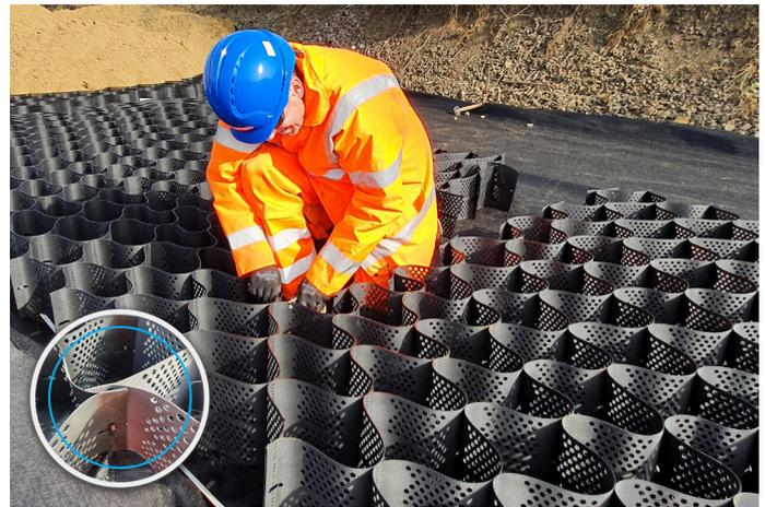
junctions located around the perimeter of an individual panel, formed during installation when adjacent panels are connected in the field, creating mechanically joined cells along panel joints. Since a primary mechanism by which geocells provide benefit is through lateral confinement of the infill, it is vital that both types of junctions remain intact during construction and throughout the design life of a project.
