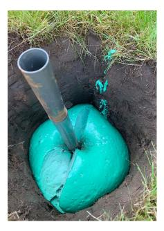
pack system is hand mixed. It doesn't need water, and a 1.8kg pack replaces three 20kg bags of concrete post mix. It therefore significantly reduces transportation costs and the risk of personal injury from manual handling.
